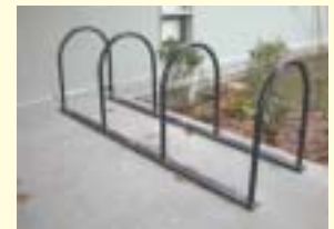
The inverted-U bike rack, whether as stand-alone units or on rails with multiple Us, make for excellent bike parking when the inverted Us are spaced at least 30 inches apart. Two bikes can use each inverted U.
