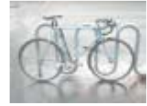
The popular wave-type rack can fully support a bicycle only when used "broadside." When used as designed, bikes are susceptible to falling down.
